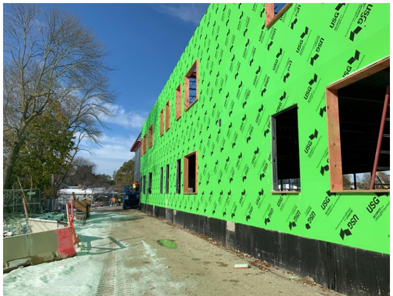
Exterior sheathing and window framing for the classroom wing.
