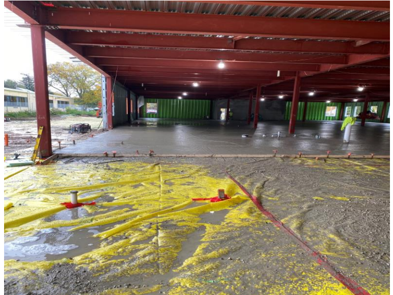
First-floor concrete slab being installed.
