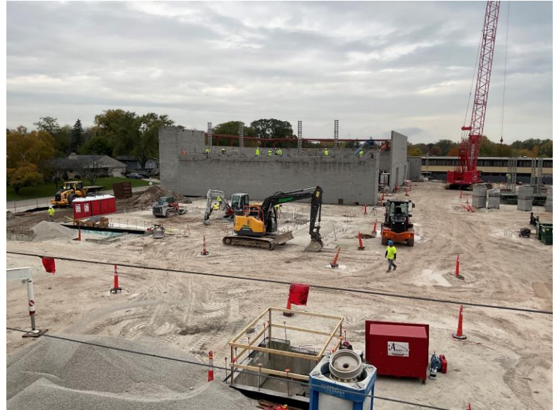
Last gym masonry wall topping out.
