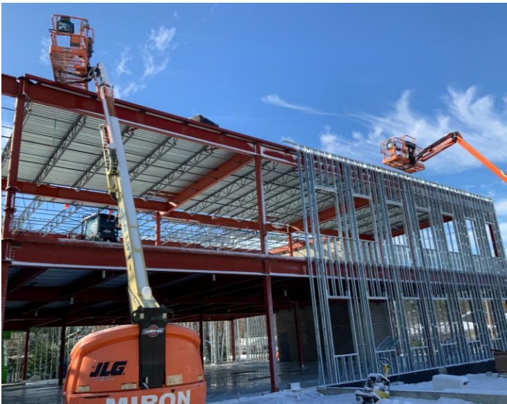
Steel roof decking installed for second-floor classrooms.
